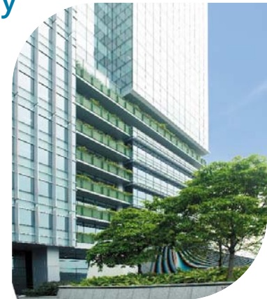
Green and Intelligent Buildings, and Energy Efficiency
